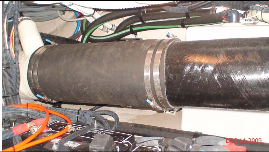
Wet exhaust system for CUMMINS engines in good condition.
