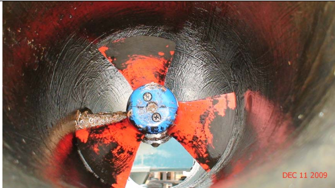
Bow thruster assembly. Monitor condition of any metal parts here and protect as necessary from galvanic corrosion.
