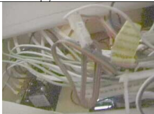
View of access to 12vDC and 110vAC electrical panels. Note that the rear of the 110vAC is not shielded.
