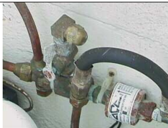
View of propane solenoid. Note capped fitting which led to the propane refrigerator. Read comment section on Propane system.
