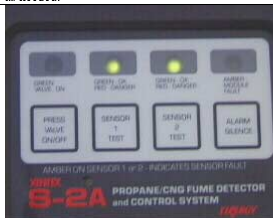
View of the Propane control system. Unit shows no fumes present in either cabins.
